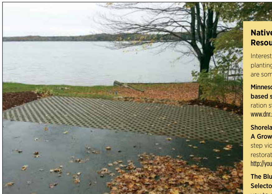
The porous paving systems installed at the Ohlrogge property capture runoff water and prevent sediment and nutrients from entering Bone Lake.
